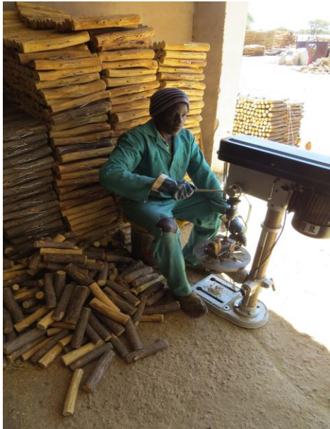
Picture 12: Independent SME operator drilling holes at pre-determined distances
