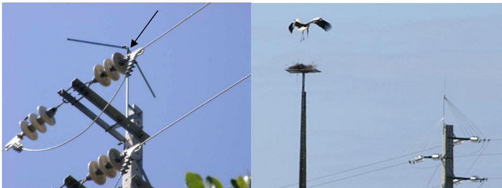
Figure 5. Distribution pole with symmetric chevron (arrow) on top as bird exclusion device (Photo: EDP-Distribution, Portugal) and dedicated nesting pole for White Stork next to distribution pole with bird exclusion device (Photo: Carlos Tiago).
