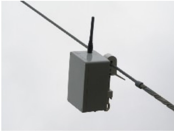
Figure 8. Bird Strike Indicator (BSI) attached to a power line. BSIs are relatively small devices that can be attached to a single wire of a power line and automatically register bird collisions based on the vibration of the wire.
