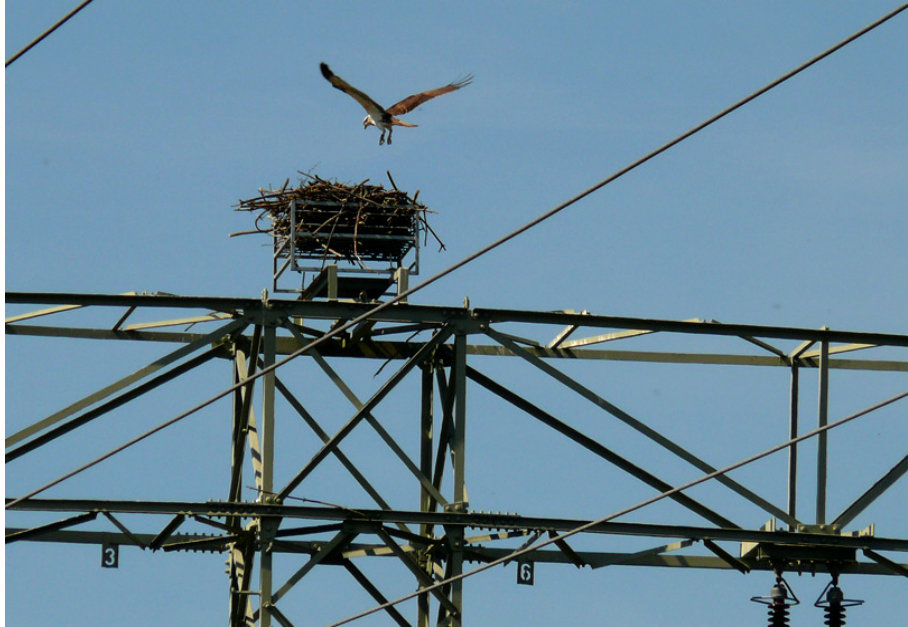
Figure 13. Nesting Osprey on artificial platform in medium voltage transmission line, Muritz National Park, Germany (Photo; Bureau Waardenburg).
