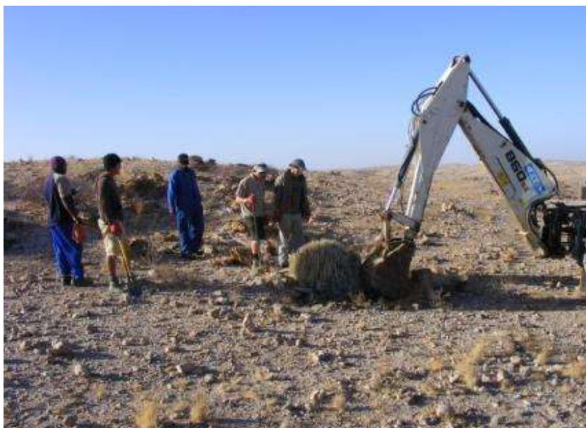
Figure 4. The excavator was used initially to loosen the soil and remove large rocks around plants (© T. Tholkes).
