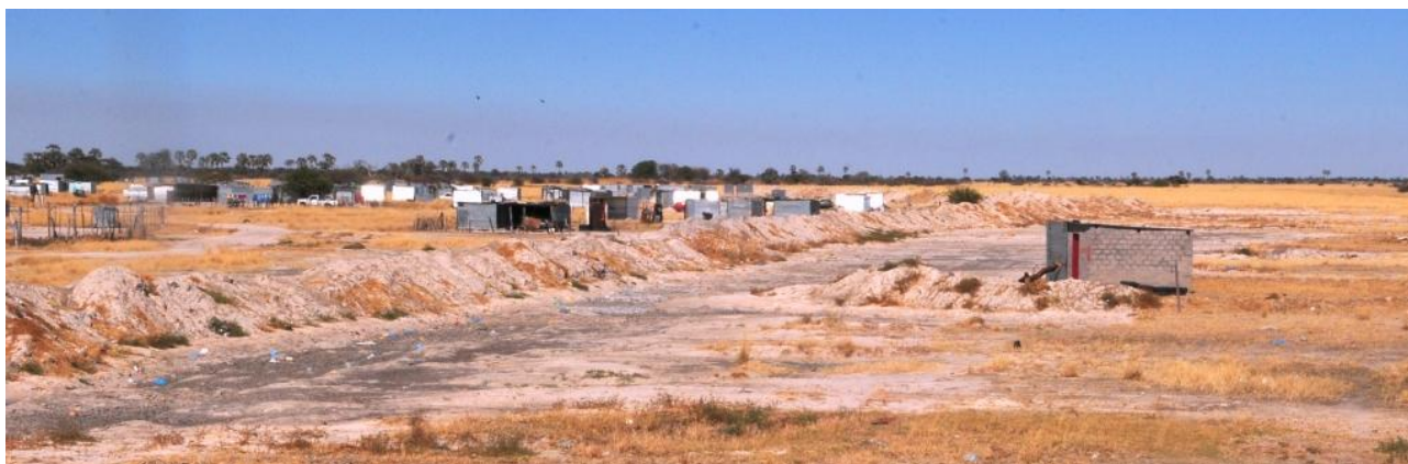
Figure 32: Bulldozed wall within oshana on outskirts of Oshakati to protect shacks (K.S. Roberts)
