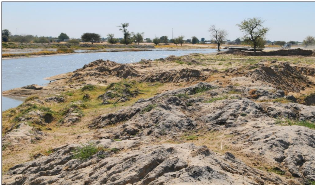
Figure 29: Bulldozed channel in Oshakati, destroying the natural margins. K.S. Roberts
