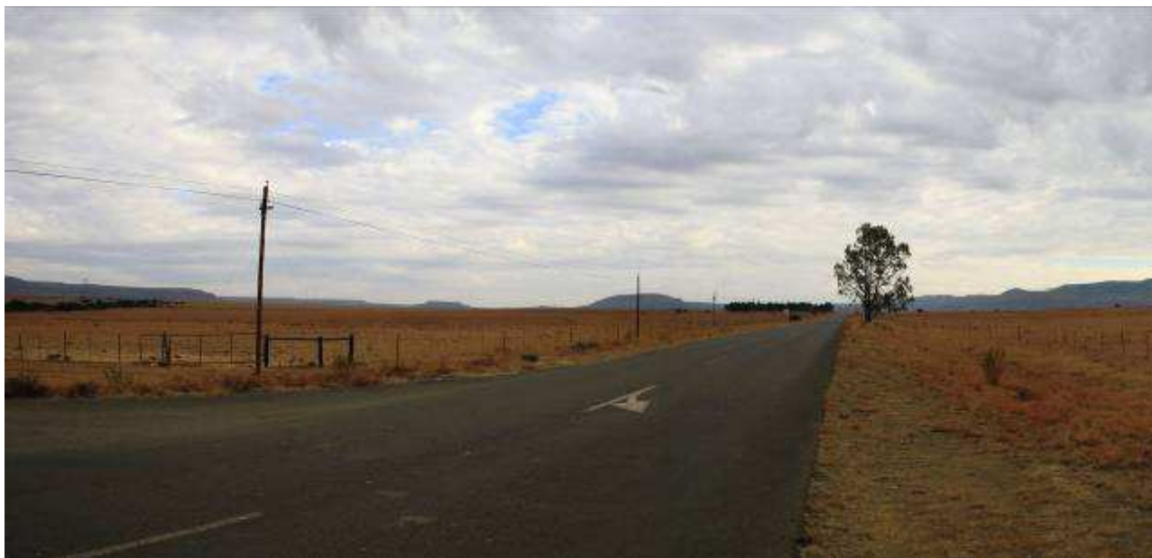
Figure 6.11: View northwest towards facility from R397 just outside Sterkstroom. The facility appears barely visible.
