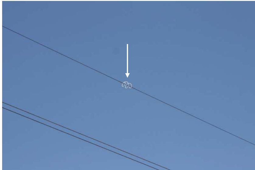
Figure 2: A coil attached to the transmission line to increase visibility for pylon sensitive bird species.
