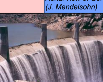
Swakoppoort Dam wall (B. Curtis)
