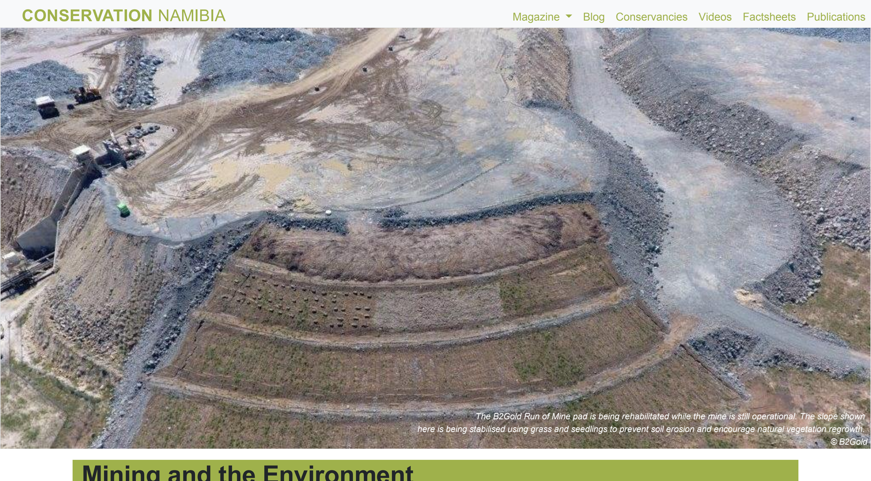
The B2Gold Run of Mine pad is being rehabilitated while the mine is still operational. The steps shown here is being stabilised using grass and seedlings to prevent soil erosion and encourage natural vegetation regrowth. © B2Gold
