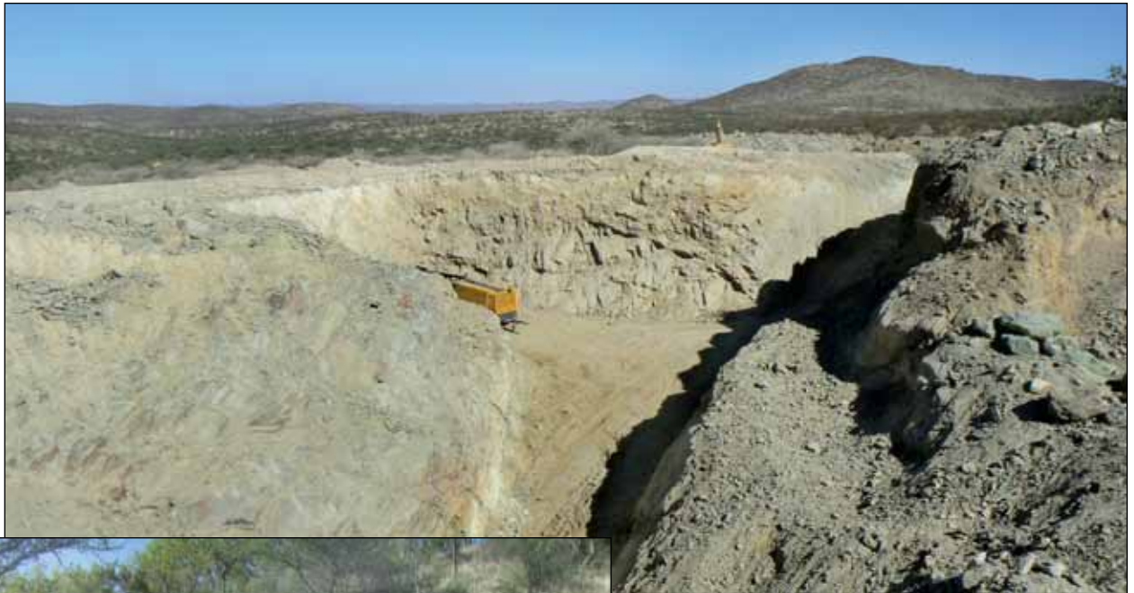
Figure 3. The Otuani open pit and box cut, in operation since 2006. The workings exploit a horizon of bornite and chalcocite ore. Robert Bowell photo, October 2010.
