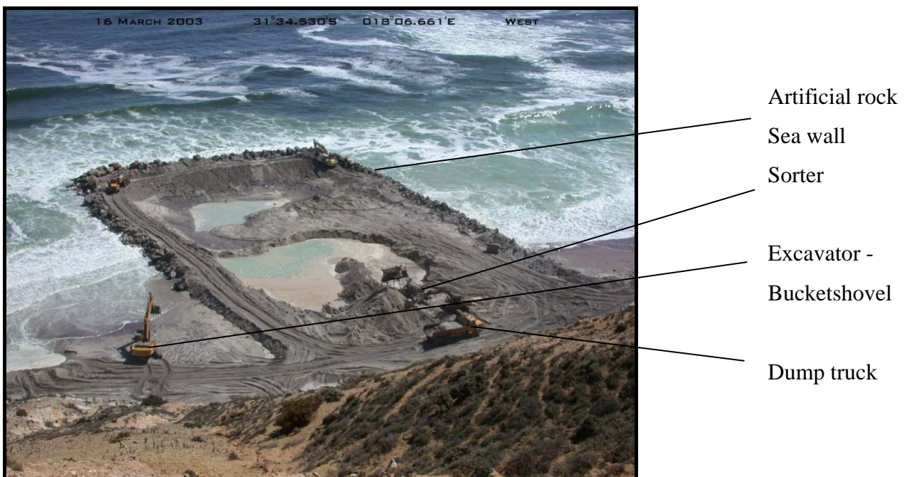
Figure 4.9 An example of a large-scale 24 hour beach mining operation.
