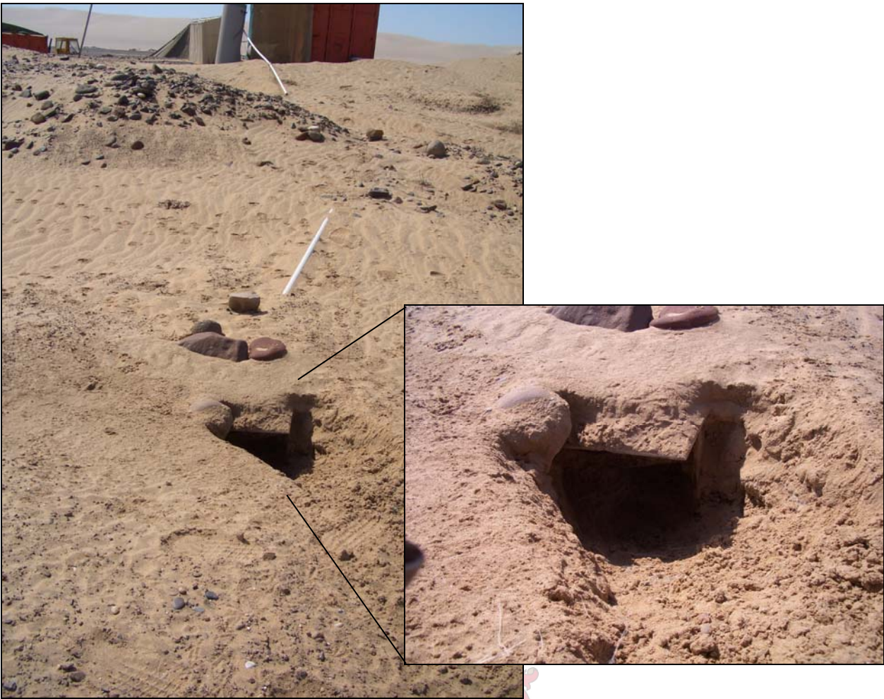
Figure 5.4 French drain on EPL 2700 (Storm Diamonds)
