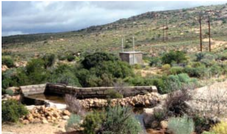
Figure 2. Filter for ephemeral spring, with injection borehole in background, Karkams (Murray & Tredoux, 2002c).
