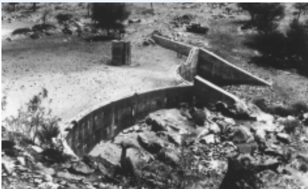
Figure 1. Early stage of sand storage dam construction, Namibia (Wipplinger, 1953).
