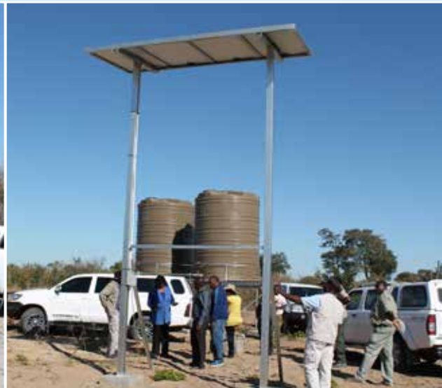
Water storage Reservoir
