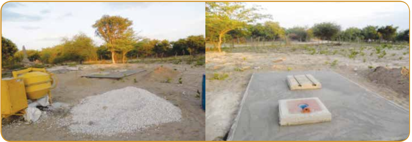
Fig. 2: Construction of septic tank at Omufitu Wekuta Community Forest.
