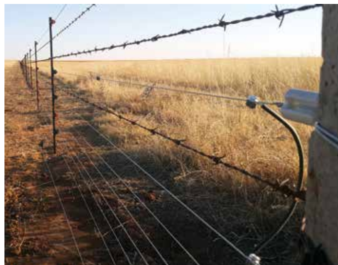
Figure 6.6. The electrification of an existing fence generally increases its effectiveness at excluding predators. Electric wires close to the ground prevent predators from crawling underneath the fence. Placing wires on each side of the live wire close to the ground may prevent the electrocution of certain non-target animals. Photo: Niel Viljoen.
