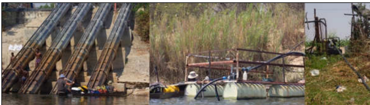
Figure 12: Typical large (left), medium (centre) and small abstractions along the Kavango River.
