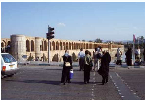
Figure 46: River bank at the Si-o-se Bridge in Isfahan (Photo: inter 3).
