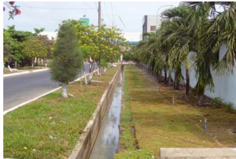
Figure 31: Open Drainage in Tra Noc (Photo: T. Fuhrmann).
