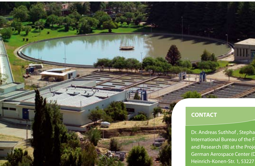
Figure 58: Implementation of infrastructure solutions (A. Künzelmann / UFZ).
