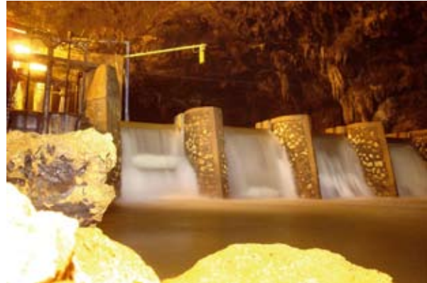
Figure 22: Existing underground dam in Bribin Cave with newly installed discharge monitoring equipment (Photo: IWRM Indonesia Project).
