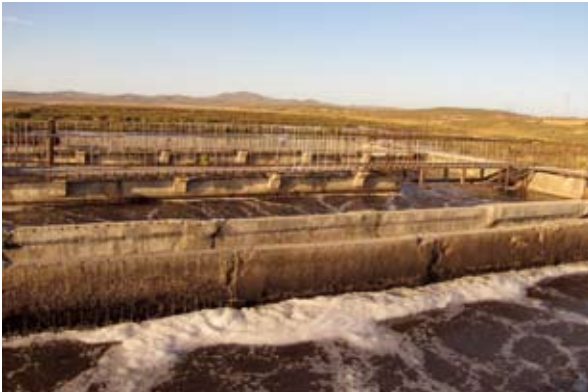
Figure 25: Old waste water treatment plant, Darkhan (Photo: D. Karthe).
