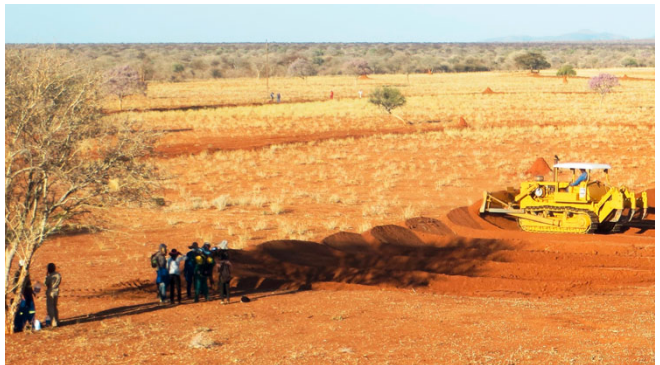
Figure 7: A ponding bank is built in September 2016 by scraping soil from above the bank.
