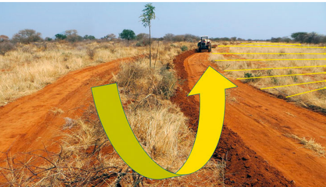
Figure 6: When grading a new ditch below the old contour ditch, the dug soil is heaped upslope so that water spilled from the upper ditch will first spread out to fill the lower ditch before spilling as wide sheet flow over the lower edge at ground level.
