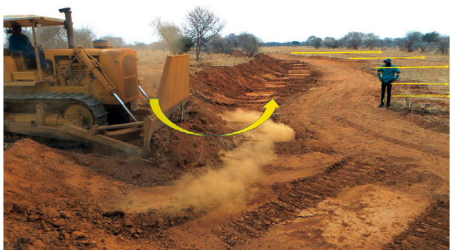
Figure 9: The bank is pushed down at its highest positions to allow spillover from ponding banks on each side to first fill the ditch below before excess water spills as wide sheet flow over the lower edge of the contour ditch.
