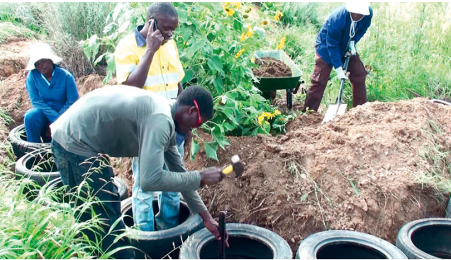
Figure 13: Old tyres are secured by steel posts to create a leaky weir.
