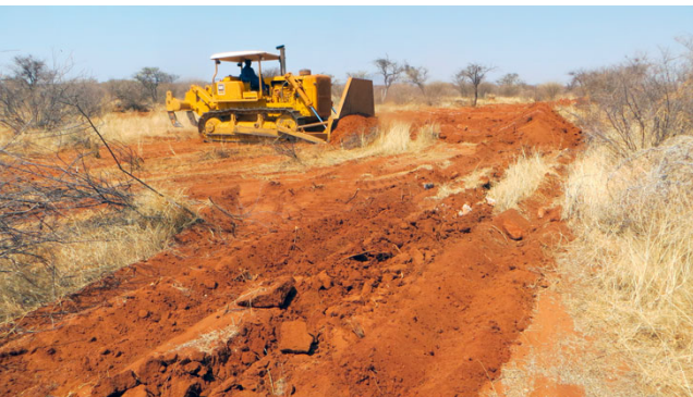
Figure 8: A ponding bank is built in September 2017 by scraping soil from below the bank.
