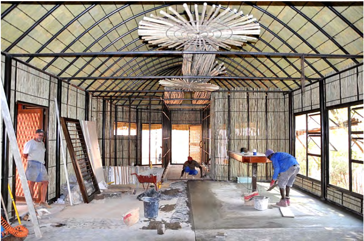
The new OPF Visitors' Centre under construction ...
