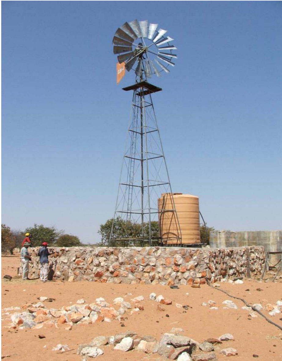
Figure 6. Successful protection wall against elephant at a water point in #Khoadi //hoas Conservancy, Kunene Region, Namibia. The wall is strong enough to keep elephants out, high enough to keep them from stepping over, and far enough from the main installations within the wall, including the plastic water tank for domestic use, to prevent elephants reaching the infrastructure. However, elephants can drink from the reservoir on the right. Photo: Olga Jones.
