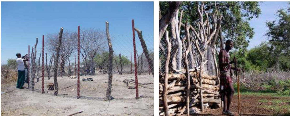
Fig. 6.1.2. Enclosures (bomas) improved with mash wire and natural logs. Photos Ruaha Carnivore Project (left) and Pat Erickson (right).
