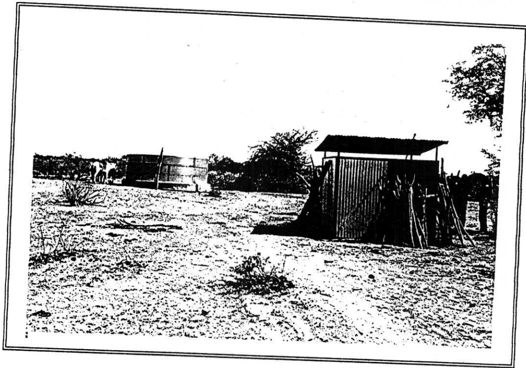
PLATE 1 Typical borehole installation maintained by Department of Agriculture, Rundu
