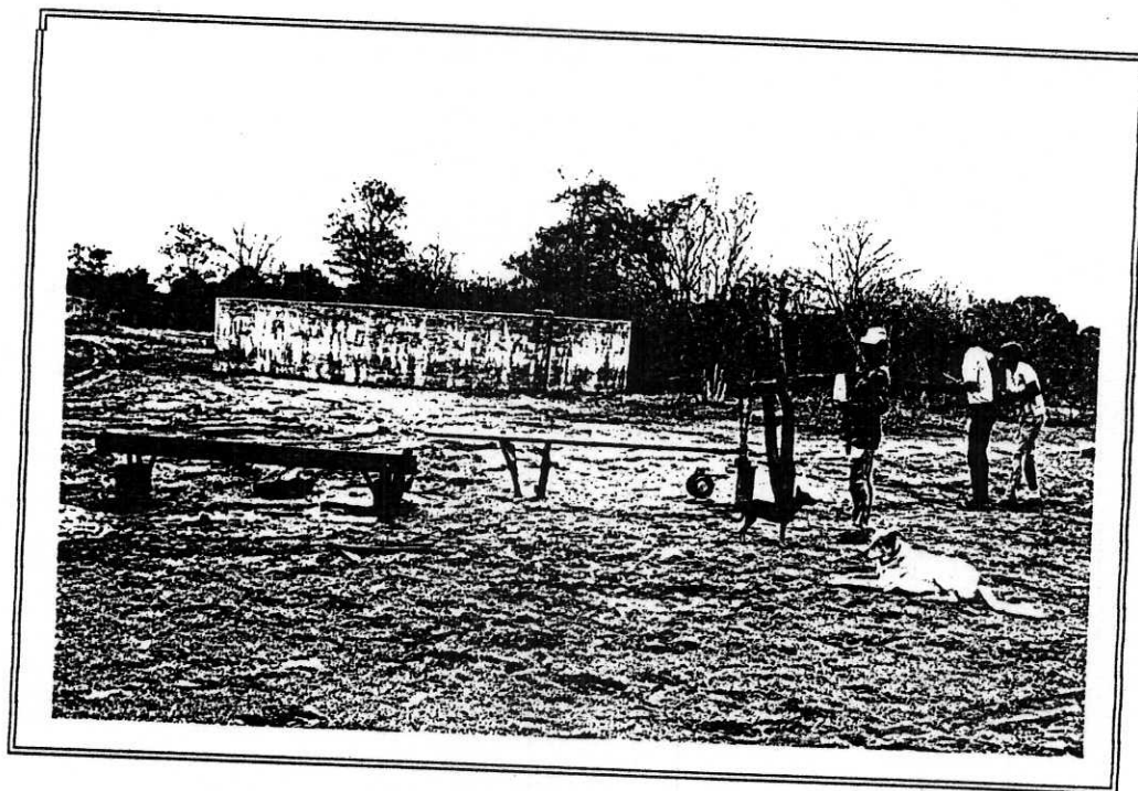
PLATE 4 Borehole with a 'wip stok' hand-pump in Kavango which has replaced the old abandoned borehole installation in the background
