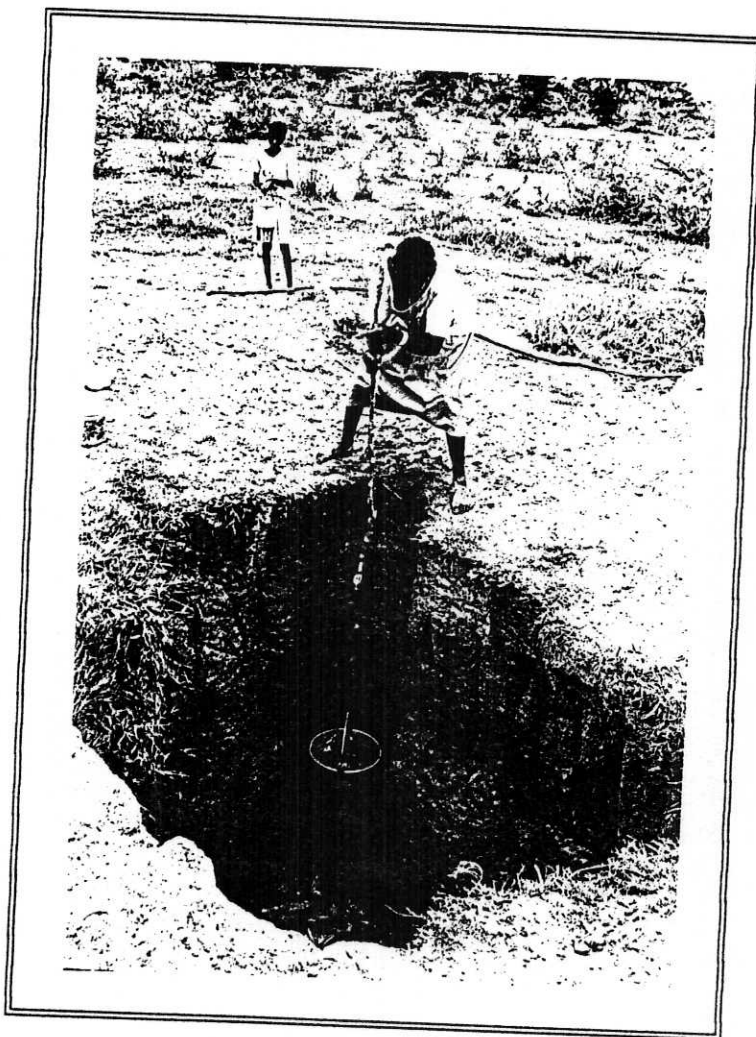
PLATE 12 Unlined well showing typical method of water abstraction for shallow water tables, Mbunya, Kavango
