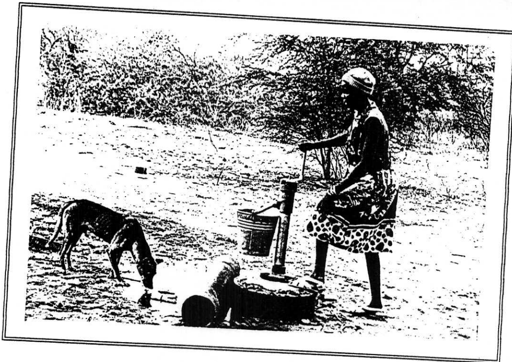
PLATE 7 'Mono' hand-pump installed by Department of Agriculture, Kavango
