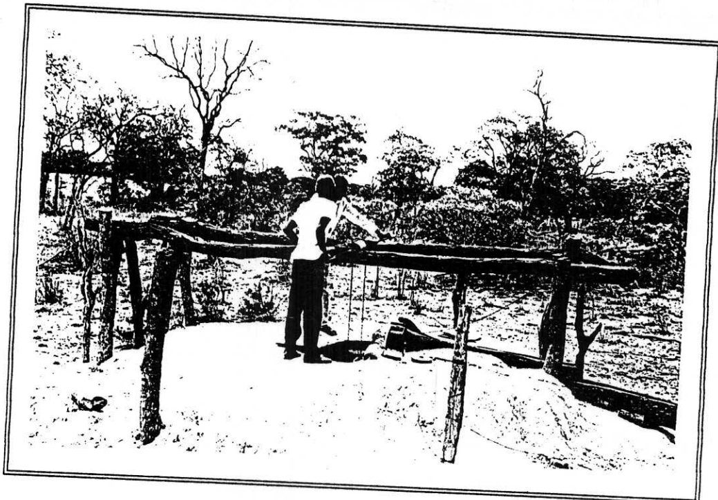
PLATE 11 Typical surface installation for the deep wells in Mbukushu
