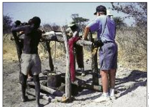
Hand-dug well within the Main Shallow Kalahari Aquifer (Oshikoto Region). The groundwater is saline and only suitable for livestock watering.
