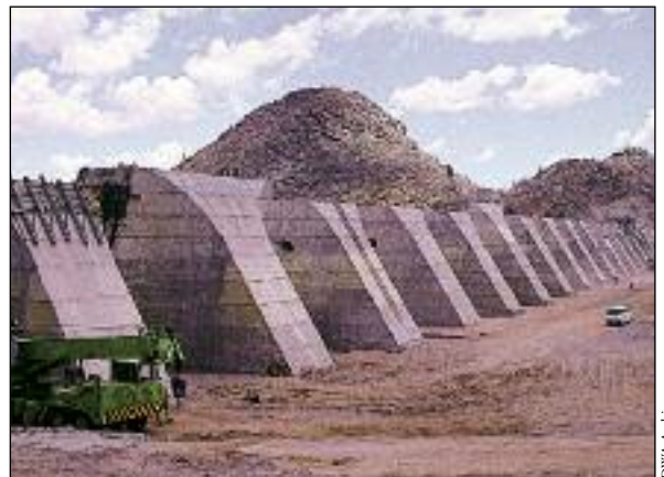
The Otjivero Dam main wall under construction
