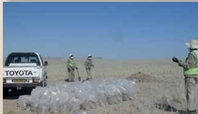
Soil polluted with oil is placed in plastic bags and removed to the skip on site for disposal at the Walvis Bay hazardous landfill.
