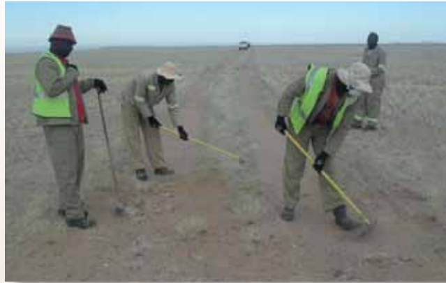
There's nothing scientific about rehabilitation work: it involves manual labour, using tools such as rakes, spades and hand picks to remove the evidence of disturbance from the surface substrate of the exploration areas.
