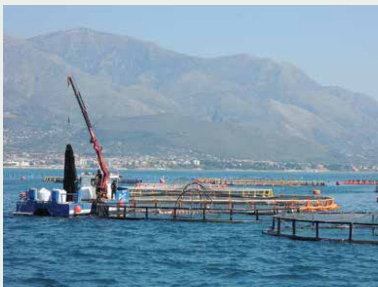
Changing the net of one HDPE cage at the P2G fish farm
