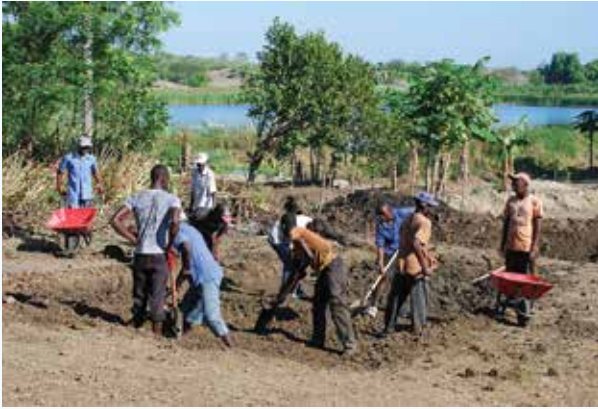
Pond digging close to Lake Robino, Haiti
