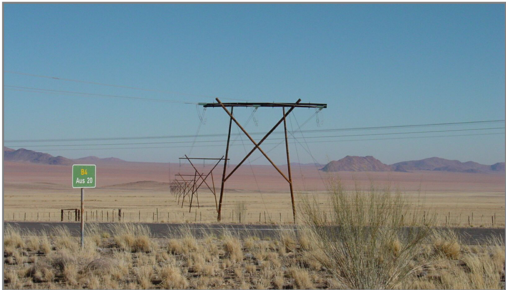
Figure 2.8: Typical 132 kV power line from Keetmanshoop to Luderitz
