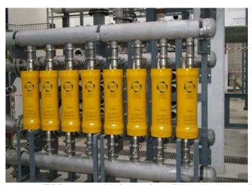
Figure 7 – ERD array with frame for 8 PX units in parallel
