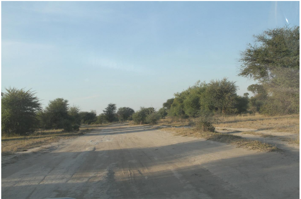
Plate 1.17: Potential for extremely slippery sections along the D3425 road during the rainy season (December – March) on certain sections of the 35 km stretch between Ncaute and the location 18^{\circ} 36'' 08.51'' S, 19^{\circ} 42'' 02.69'' E, along the Omatoko Ephemeral River Channel.
