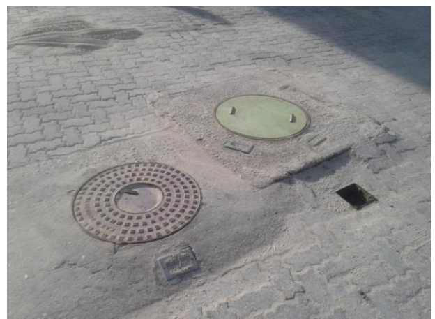
Photo 6. Underground storage tanks (1 ULP & 1 Diesel)
