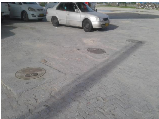
Photo 5. Underground storage tanks (2 ULP & 1 Diesel)
