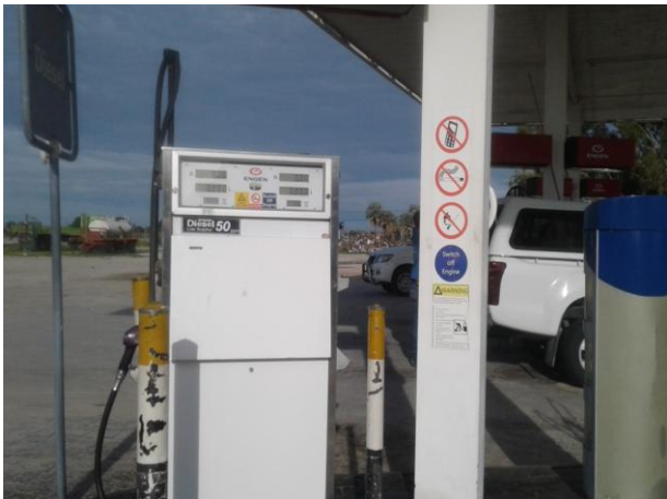
Photo 3. Single-hose dispensing point (50ppm Diesel)
