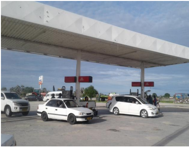
Photo 1. Existing dispensing points and canopy
