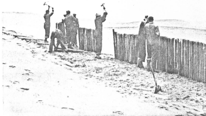
Fig. 1. Erecting a pole barrier.
