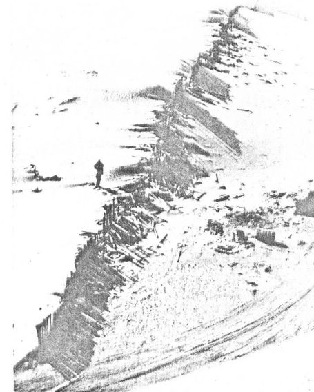
Fig. 2. Severe damage done to the barriers by strong winds.
