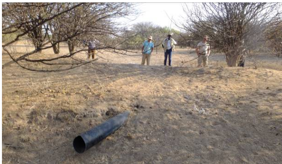
Figure 4: A pipe in a dam wall provides opportunities to pulse the release of water to favour grass growth, if fitted with a valve at its outlet.
