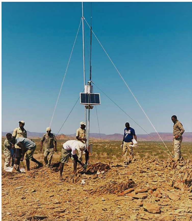
FIGURE 4 Erection of Early-Warning Tower, Anabeb Conservancy, April 2020.
