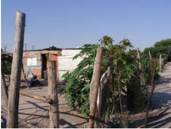
Corrugated iron structure in Ndama
