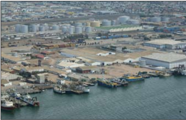
Above: The main port in Namibia, Walvis Bay Harbour in Erongo region (© N. Cadot)
