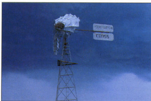
Fig. 2.20 Borehole pump at Khowarib. Courtesy E Marais
