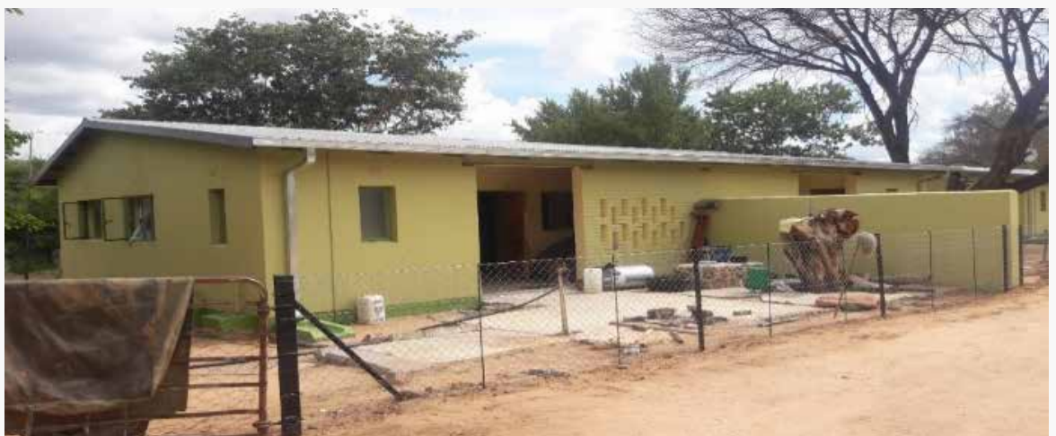
A refurbished staff house at Onyoka in Waterberg Plateau Park.
