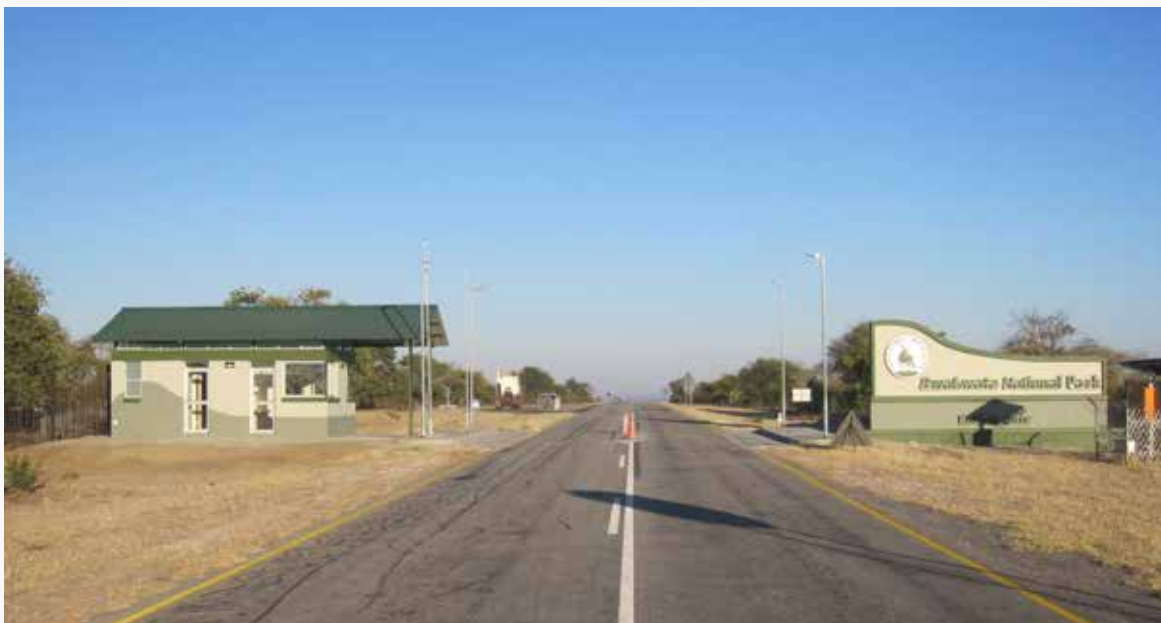
Construction of new entrance gate to the Bwabwata National Park.
