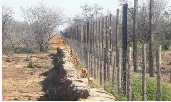
Electrified 20km section of the Waterberg game proof fence.
