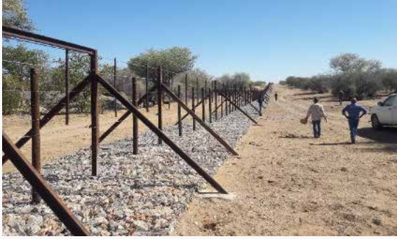
Completed Kaross Section of Etosha National Park boundary fence.
