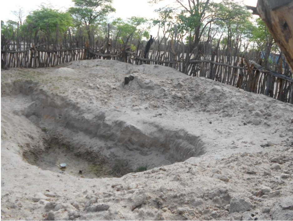
Figure 14: A shallow hand dug well
