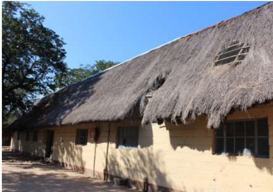
Figure 18. A community hall at Omega (Bwabwata National Park) thatched with a mixture of kasisi and mahengehenge ( Cymbopogon caesius and Hyperthelia dissoluta ) in the 1980's. Except for loss of material due to improper maintenance, the condition of the thatch is surprisingly good.
