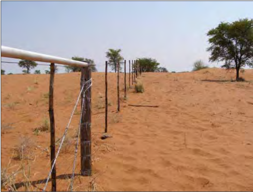
Livestock-proof fencing (designed only to constrain the movement of livestock)
