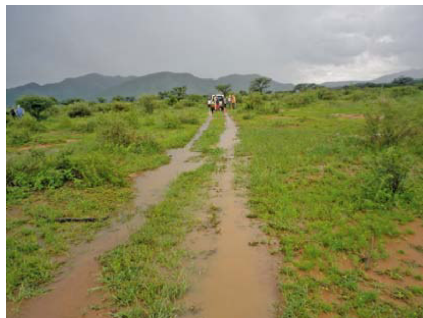
Figure 12. The track is capturing almost all of the sheet flow from the left side and the lower, right hand side of the photograph is now effectively dehydrated by the "track creek".
