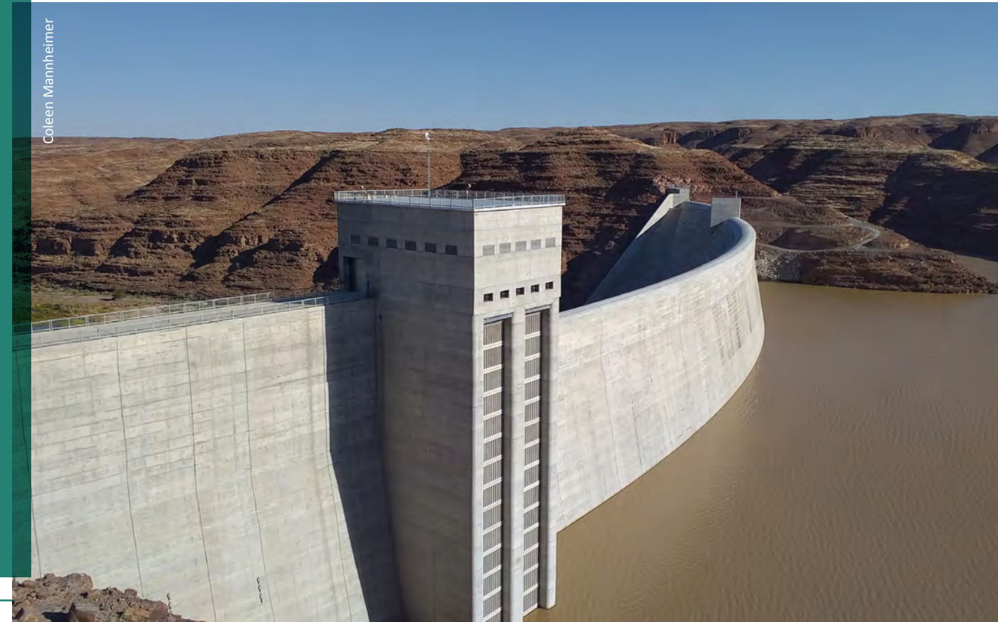
The newly completed Neckartal Dam impounding water
