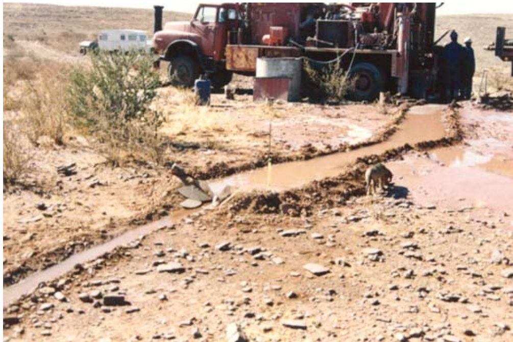
Figure 11: WW34684, drilling in progress
