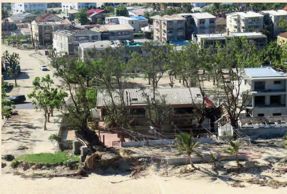
Damage to coastal infrastructure in Beira after Cyclone Idai [image courtesy of Celia Macamo]
