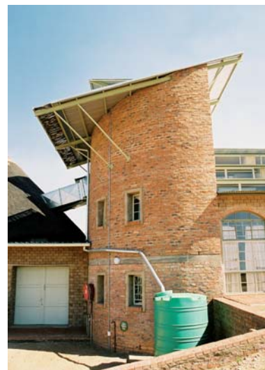
LEFT: Recycling of swimming pool backwash water can result in water savings of 20 - 30%. RIGHT: Simple rainwater harvesting techniques, as demonstrated at the Habitat Research and Development Centre (HRDC), provides abundance of spare water capacity for various uses.
