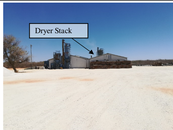
Photo 6. Tile grout factory and dryer stack
