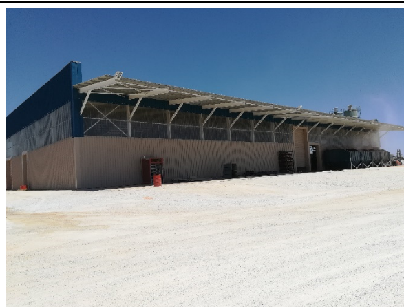
Photo 2. Brick manufacturing building
