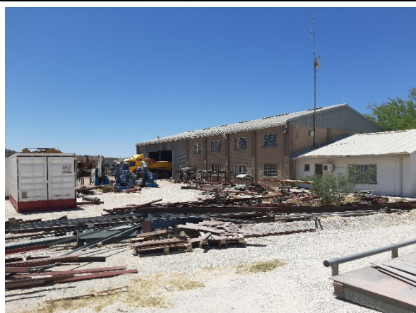
Photo 15. Maintenance storage yard and workshop
