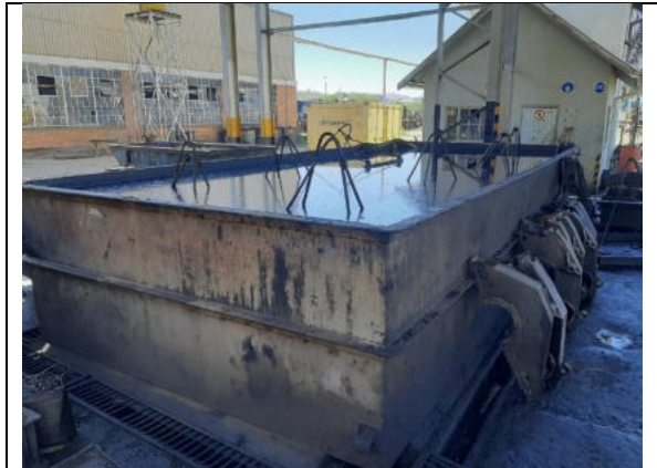
Photo 4-8 Waste oil tank
