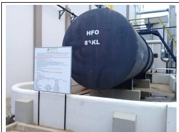
Photo 3. Tank bunding and operational signage
