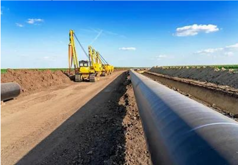
Picture 2: Image illustrating pipeline site preparation and construction (Hidenis Group LLC, 2020)
