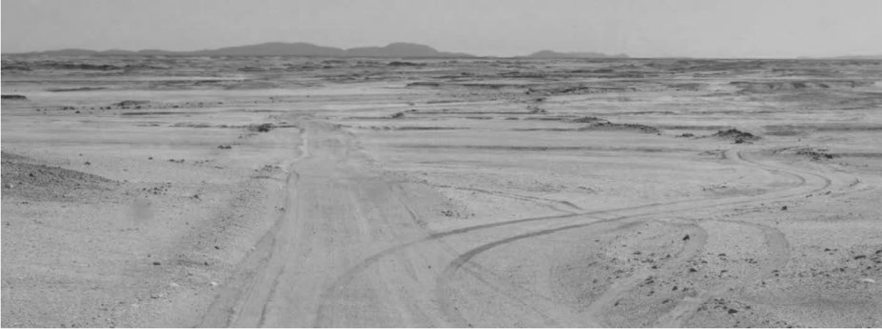
Figure 13: Shows current status of the access track to the site (AOI), the main track appears to be regularly maintained by grading
