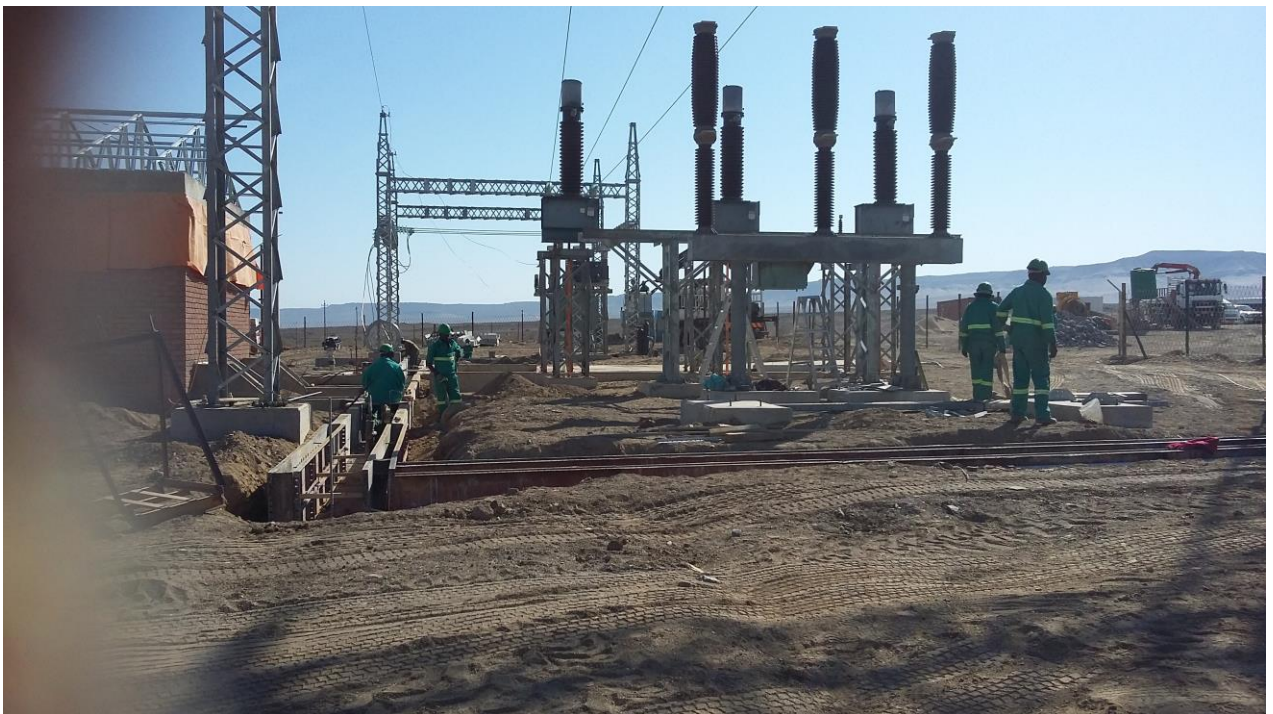
Figure 2: civil and mechanical work onsite.
