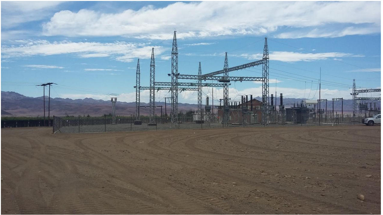
Figure 4: At the completion of the Substation Expansion project.
