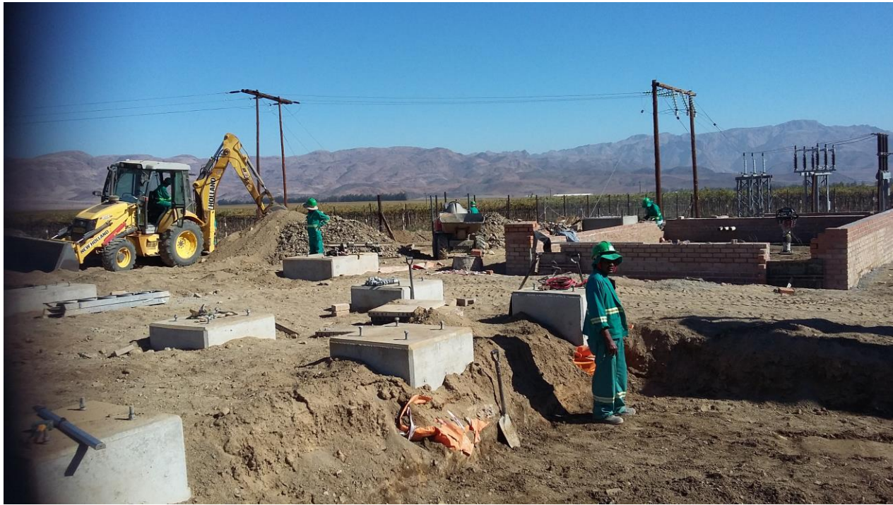
Figure 1: Foundation columns in place and vineyard in the background.
