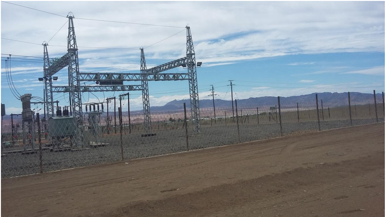
Figure 3 : Mechanical work completed.
