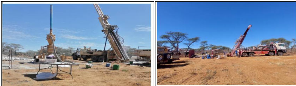
Figure 2-4: A drill rig on an EPL in the Omaheke Region (Resilient Environmental Solutions, 2022)
